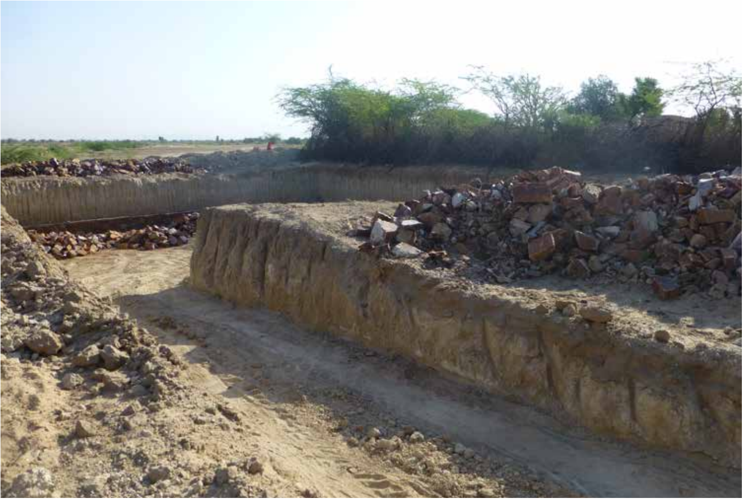
Figure 2 Earthworks at Plantation, Bagariyon ki dhani , May 2015
