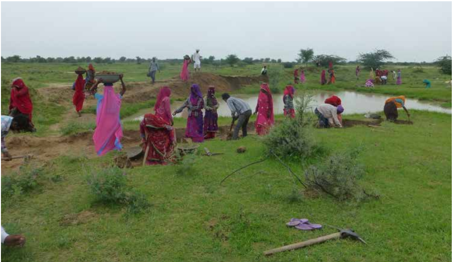
Figure 6 Work in progress in Bansi nadi, Kankaria September 2015
