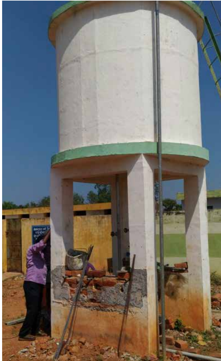
Figure 9 . Repair work at Thervoy overhead tank, Feb 2016
