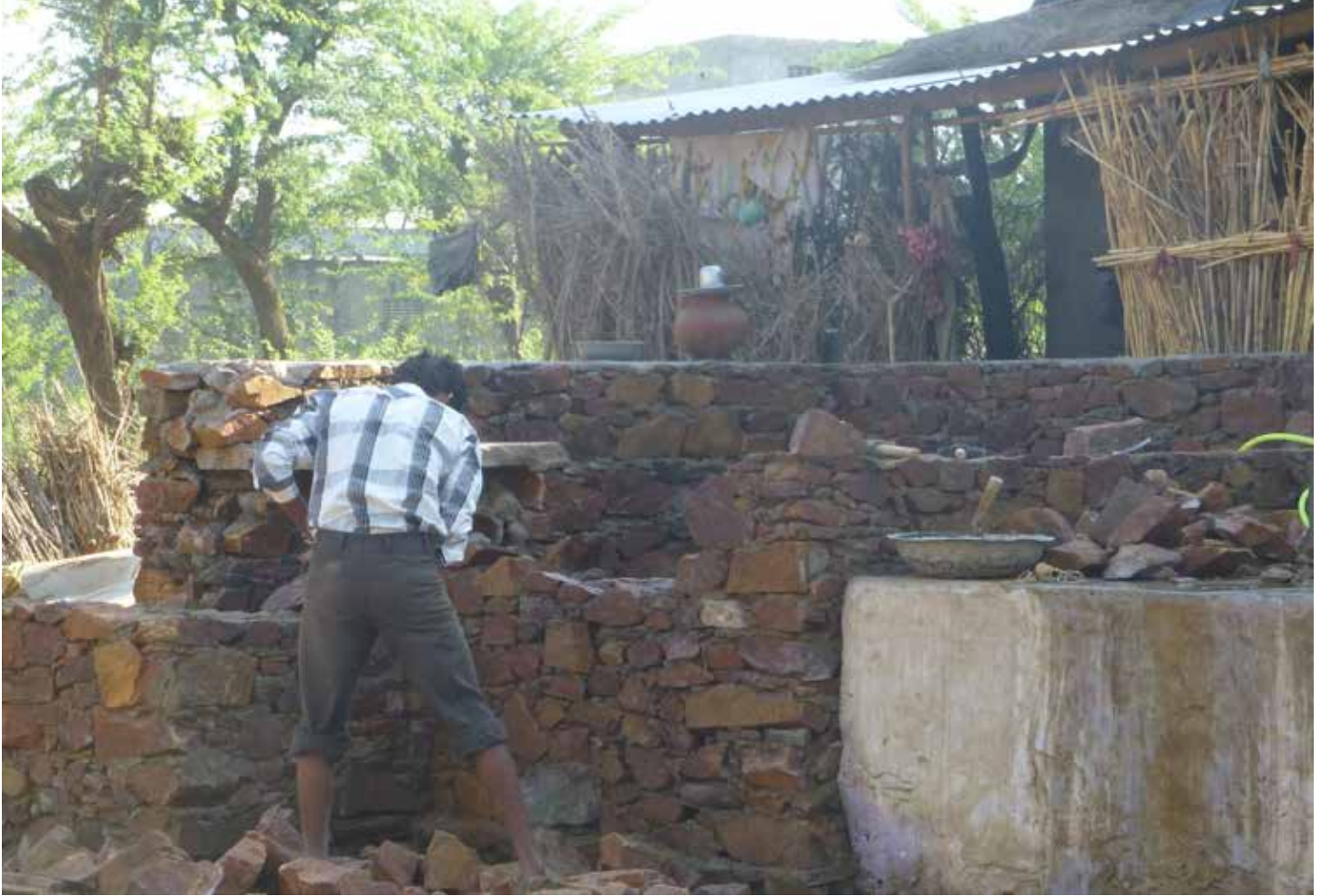
Figure 13 Construction of water storage tank at Shayam Lal's home ,Kotri
