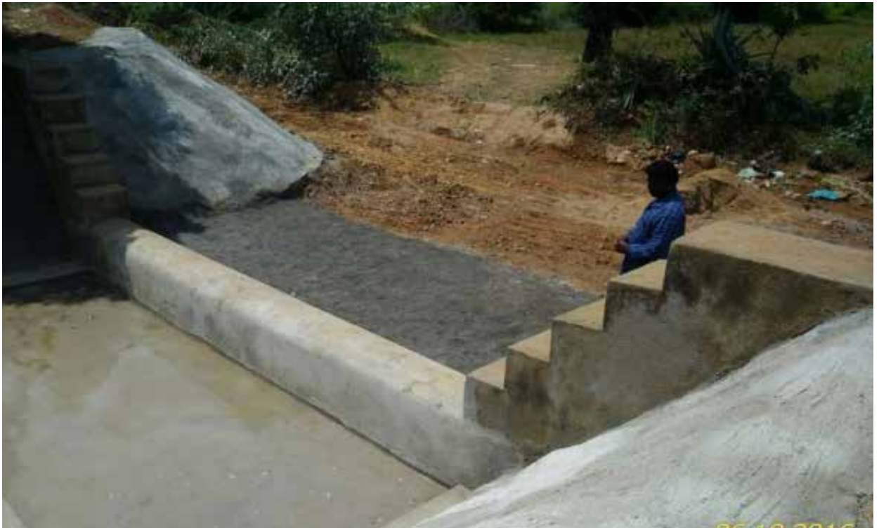
Fig 4: Palaiyathan Eri Work in Progress
