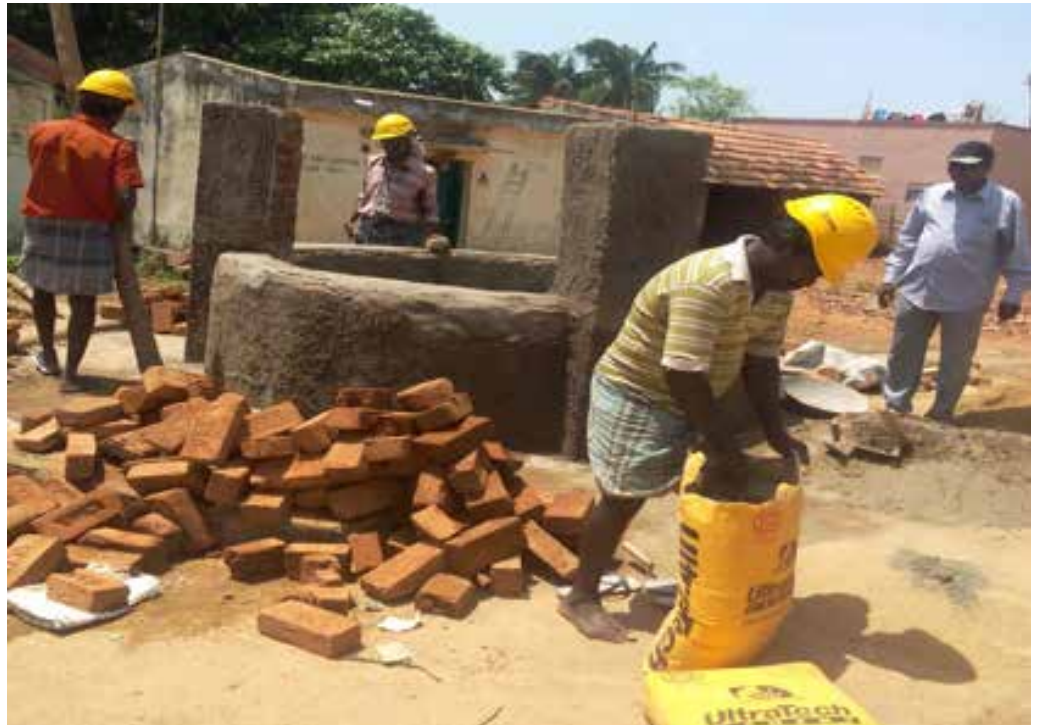
Fig 3: Kollanoor Well Renovation
