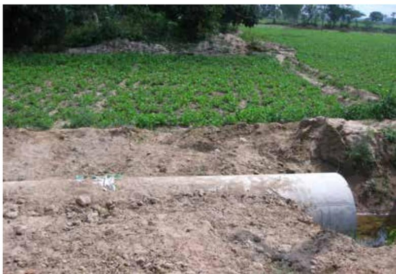
*Culvert inserted in the feeder channel to Sivan Koil Kulam*
