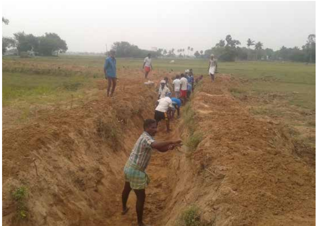
Figure 18 : Mukkarampakkam Eri Sluice No 2, during restoration
