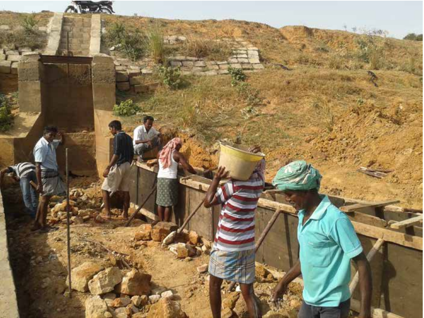
Figure 15: Mukkarampakkam Eri Sluice No 1, June 2014
