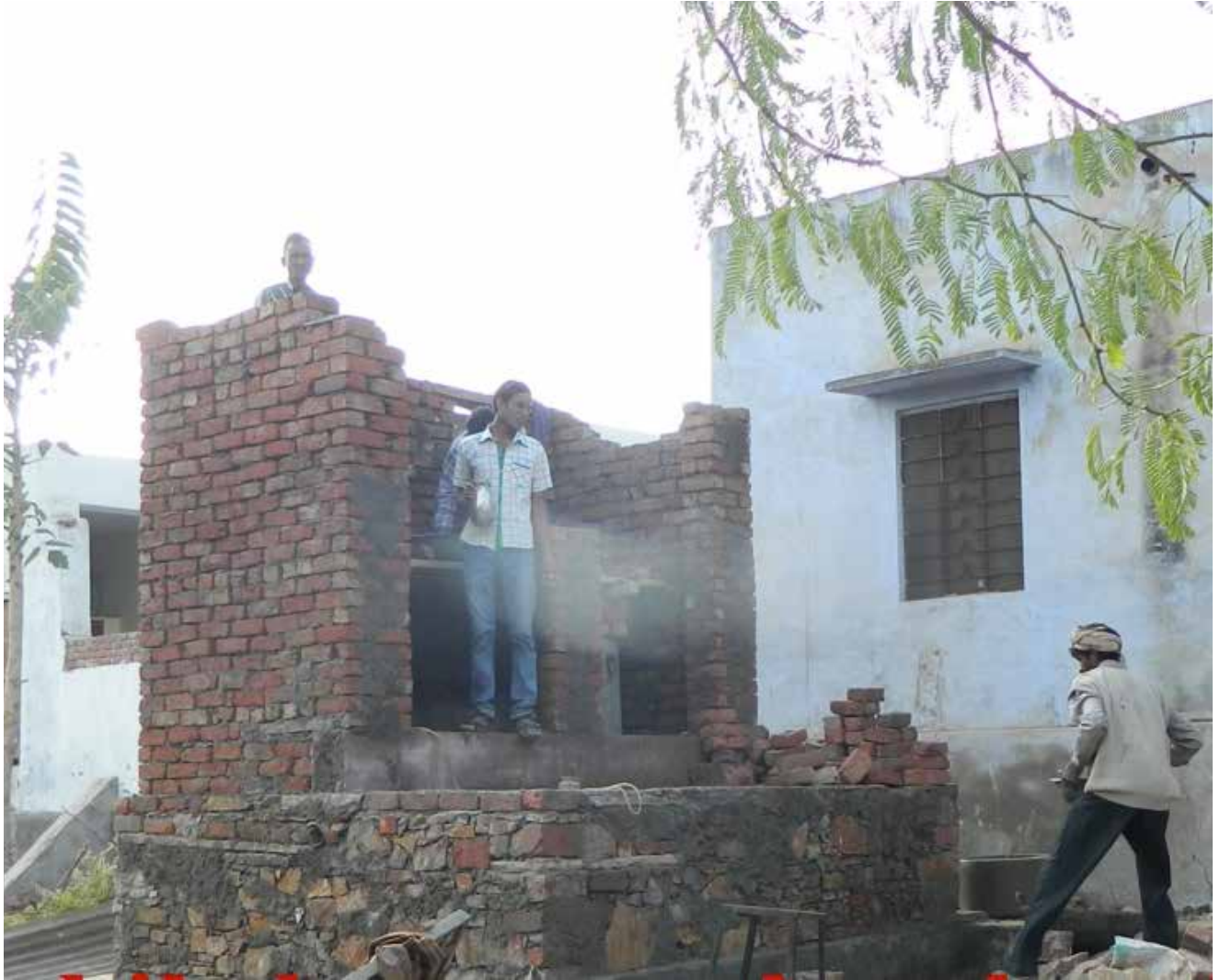
Figure 22 : Construction of toilet, Manthan girls' school
