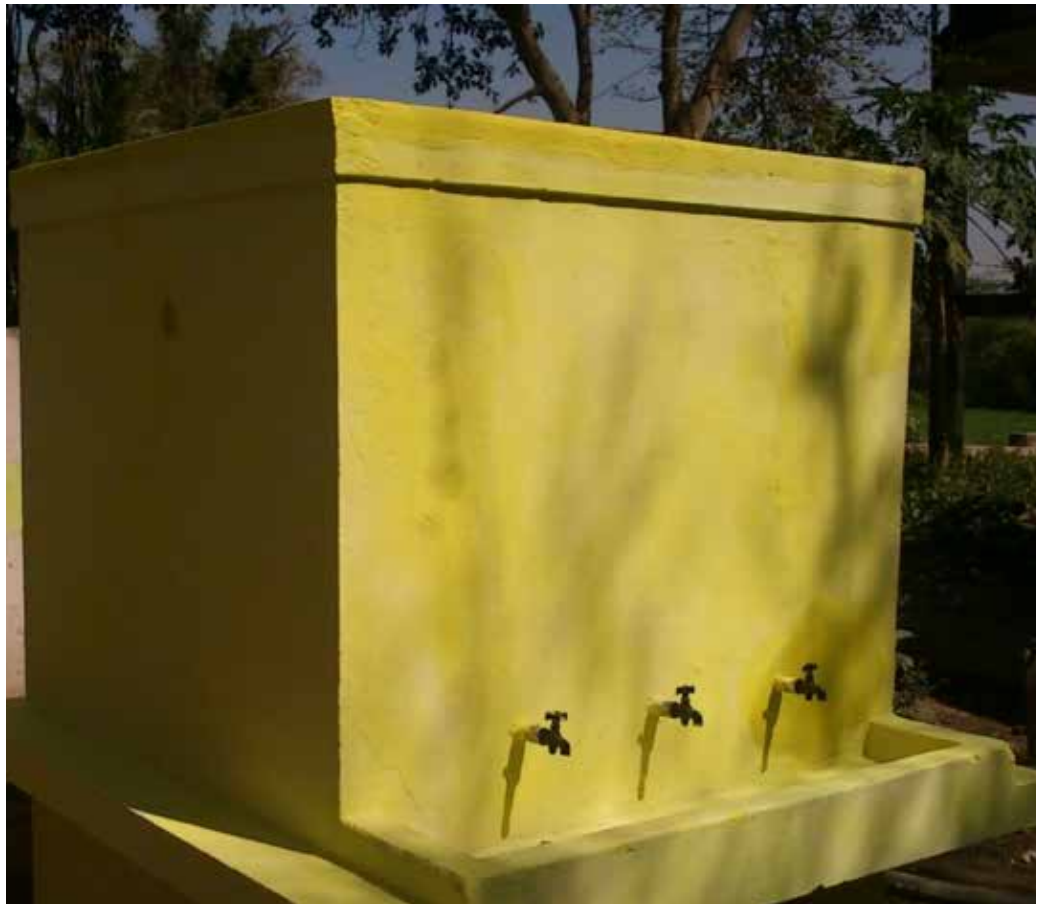
Figure 19 : Cleaned and repaired tank in Kizhkarumanur Primary school
