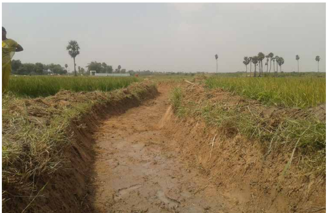
Figure20 : Mukkarampakkam Eri Sluice No 2, after restoration
